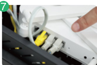
Step7: Connect LAN cables to router
