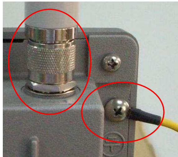
Figure 7 – secure antenna and grounding cable
