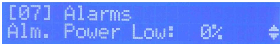
Fig. 5.40 – Alarm power Low menu
