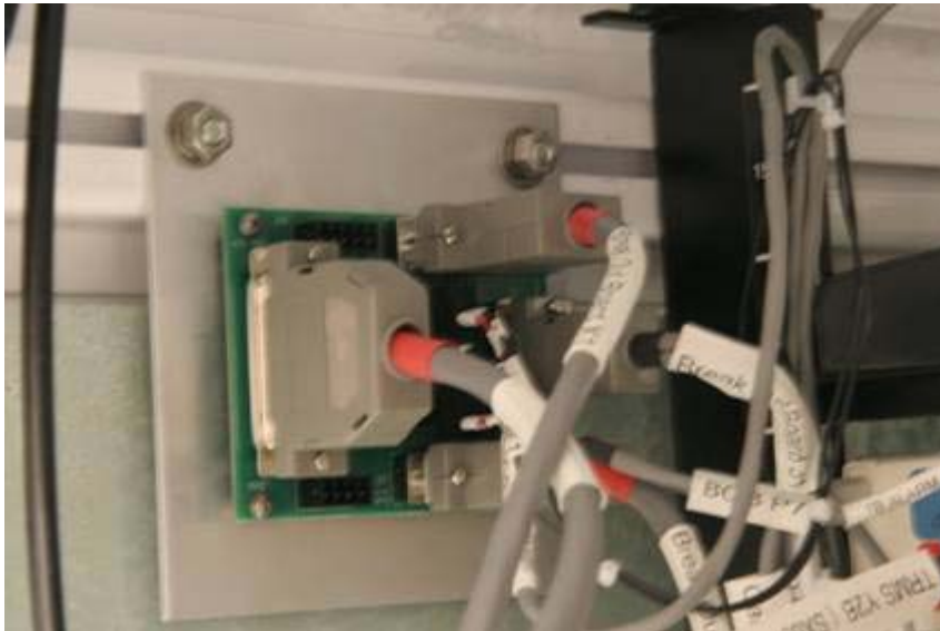
Figure 3-32 Break Out Board Installed in DRU
