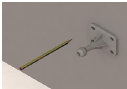
Figure 7: Marking the drill pattern
