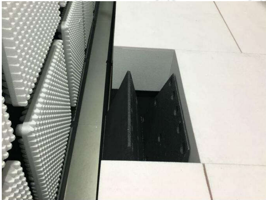
There are absorbing materials under the ground
