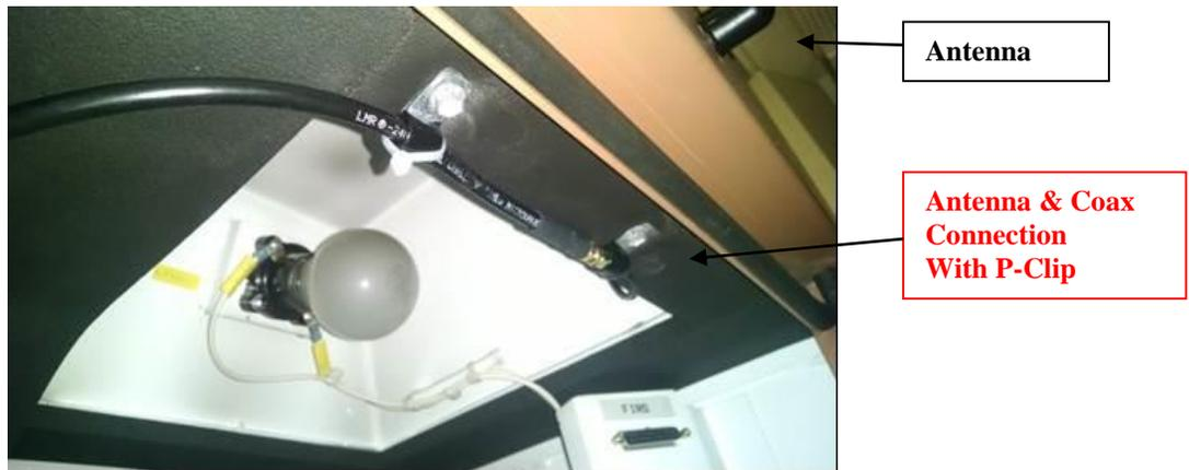
**Figure 4.6: Antenna Cable P-clip and Coax Support**
