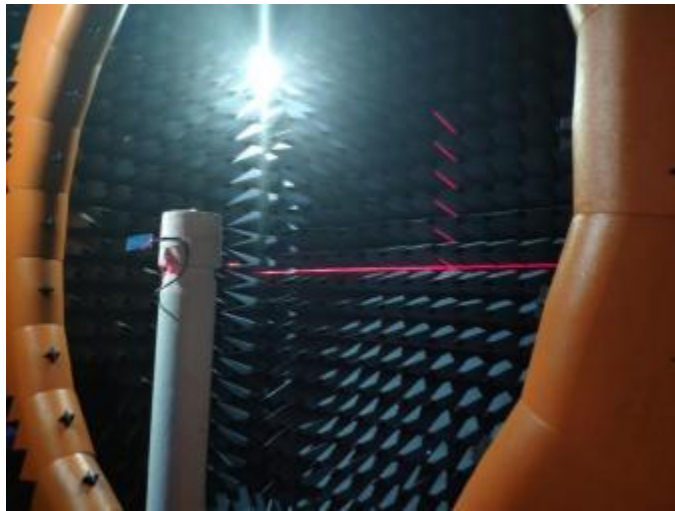
7*4*3M 3D microwave anechoic chamber
