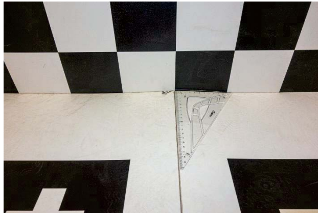
Finding a line perpendicular to the wall
