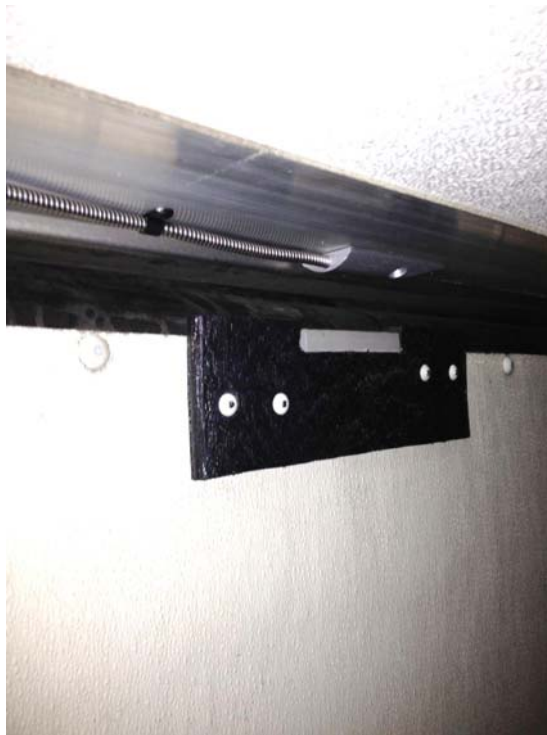
Door switch mounting on the inside of a swing door.
