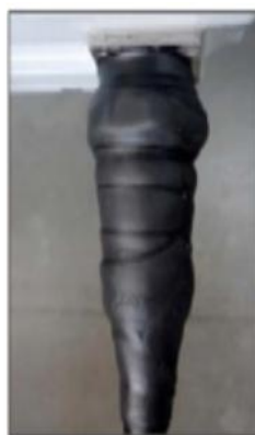
Wrap three layers of waterproof mastic
