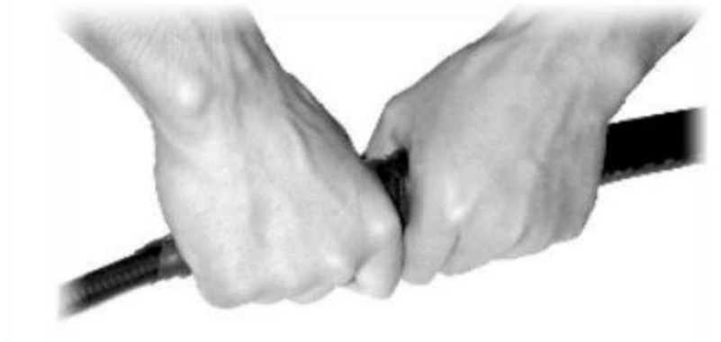
Figure 3-4 Compacting the waterproof mastic
