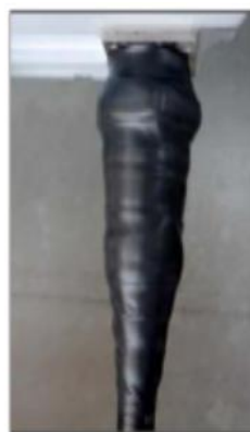
Wrap three layers of electrical tape
