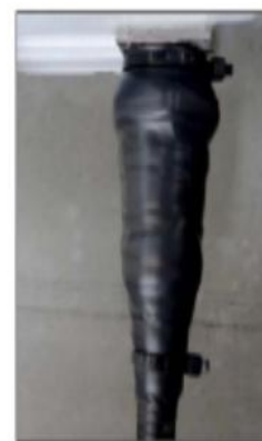
Secure both ends with cable ties.
