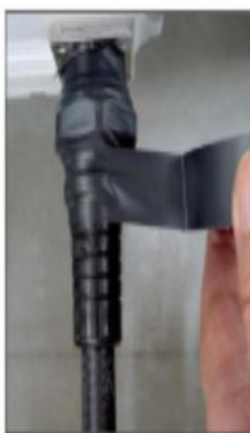
Wrap one layer of electrical tape.
