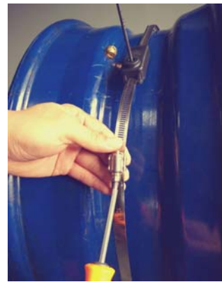
3、 Pre tighten steel tie screw
