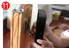
Protect cable before fixing emitter.
