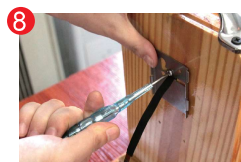
Tighten screw to fix steel board.
