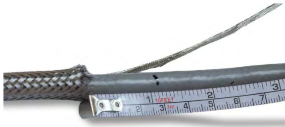
Figure 2-32: Marking the Cable Jacket
