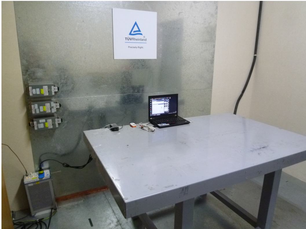
Photograph 6: Set-up for Mains (Front View)
