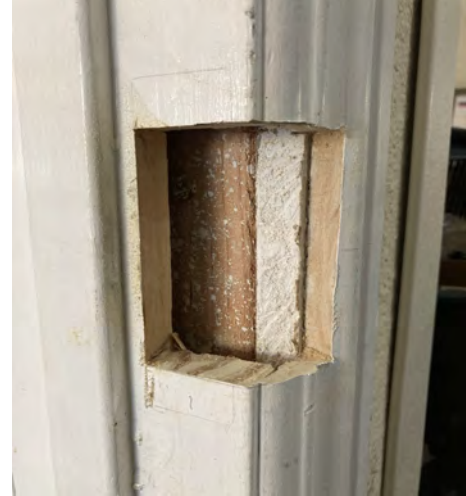
Cutout Frame using Oscillating Tool
