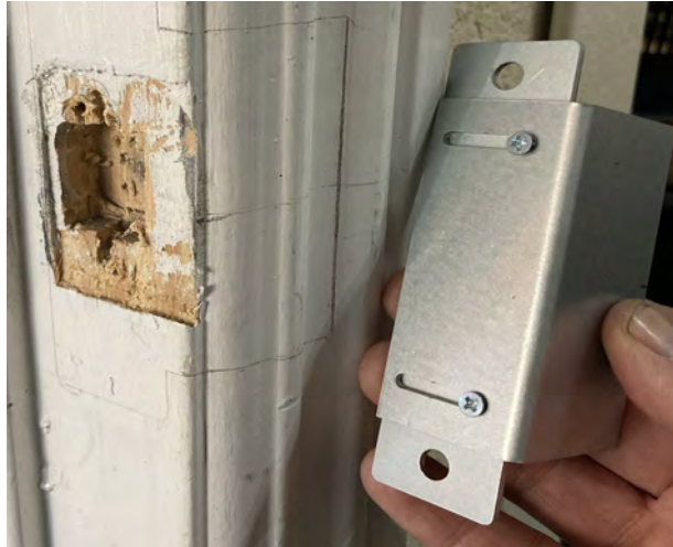
Mark Cutout with Guide (Adjust as Necessary)
