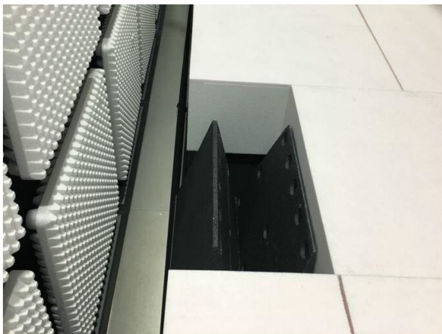
There are absorbing materials under the ground
