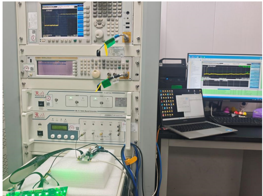
Radio Test Setup View
