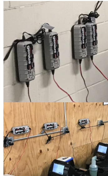
Figure 15 Examples of Charger Mounting Orientation
