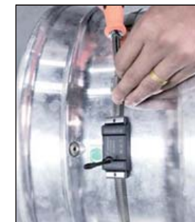
⑤Tighten the steel tie screw
