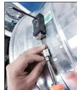
④nstalling non-slip rubber pad
