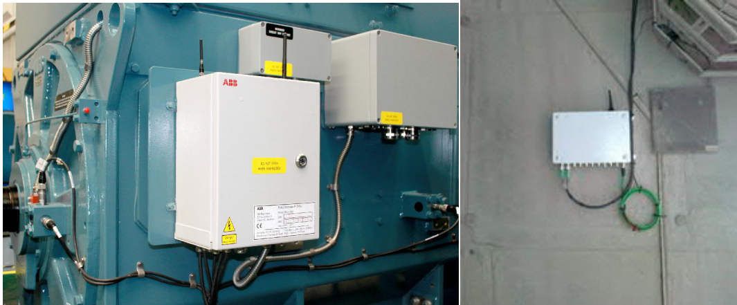
Examples of Mounting DAU on a Machine
