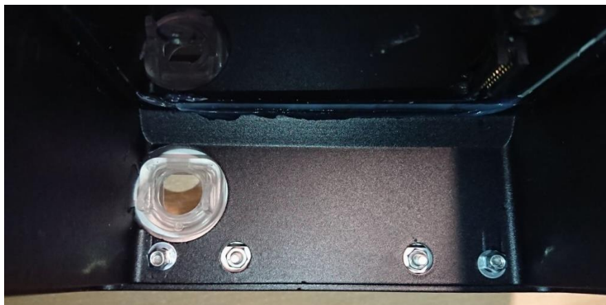
Internal view of the boards assembly place
