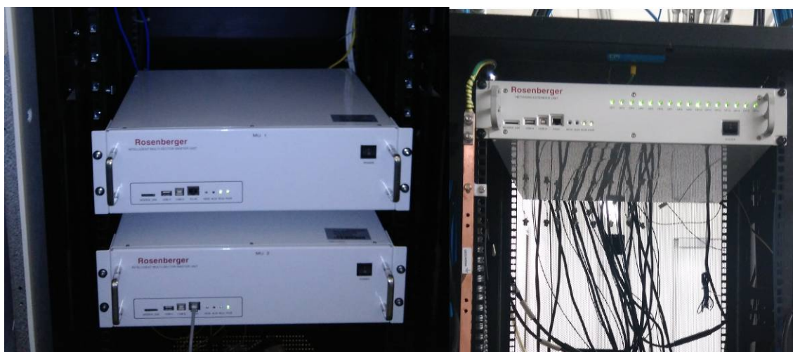
Figure 17 Installation of IM2U and NEU
