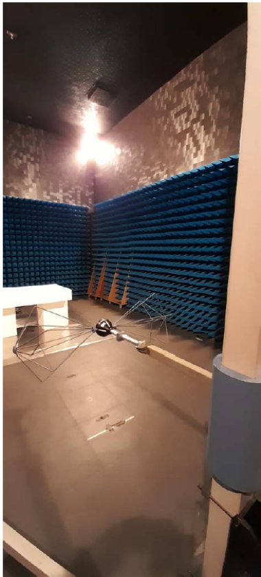
Photo antenna tower :
