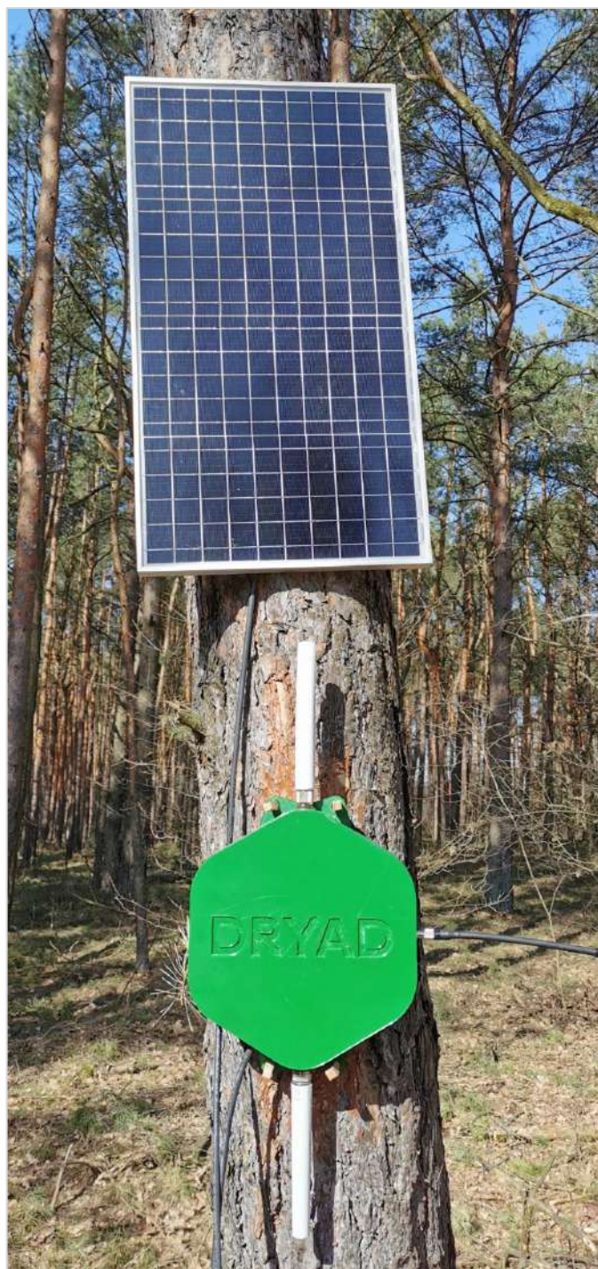
Solar panel attachment completed
