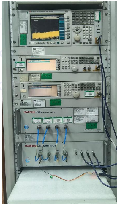
Photo of Setup for Conducted Measurements
