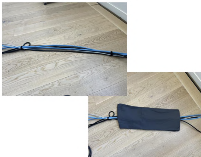
Figure 45 On the left, bundling cable. On the right, covering them.
