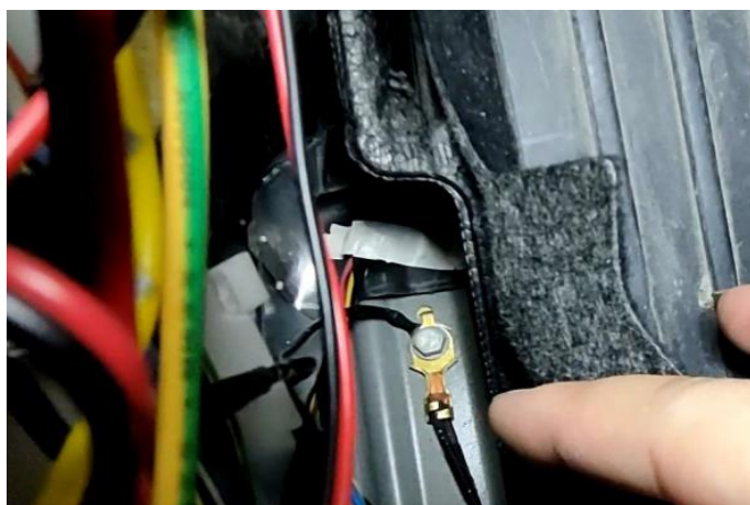
(4) 在主驾驶脚踏旁边接地线。接好之后测试把手，把手工作正常即可恢复车门饰板 Ground wire next to main driver's foot. After connecting the handle, test the handle to restore the door trim panel when it works normally
