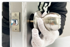
1.Install the front lock and pass the tail measure through the square rod hole of the lock body
