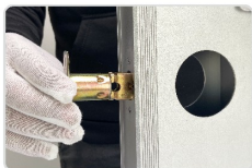
1.Mounting lock body
