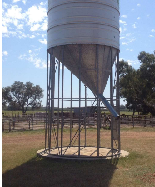
Figure 3: Example of silo with an asymmetric cone
