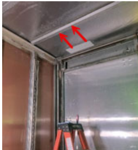
IU Direction of Force for Removal
