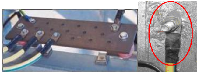
Figure 2-5 Ground Connection
