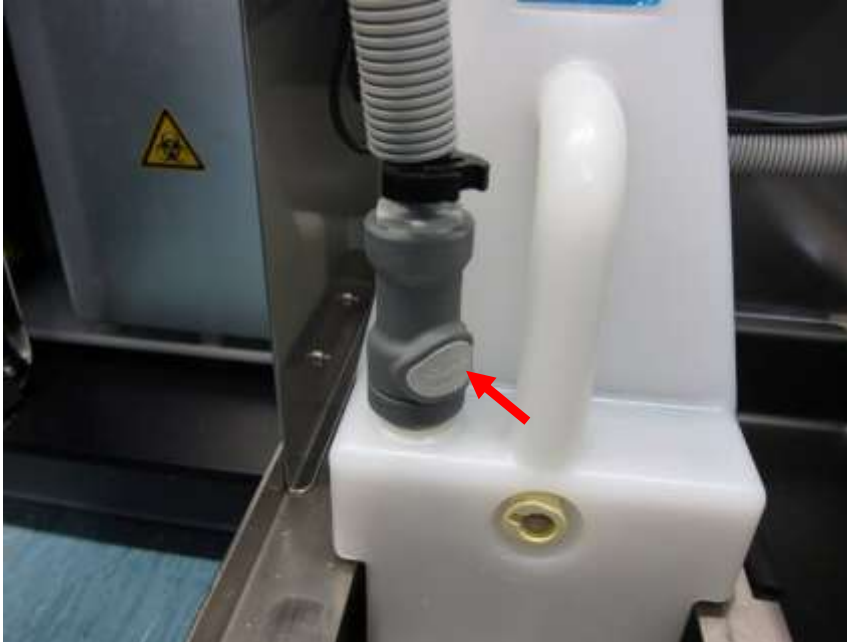
Figure 12-12: Direct plumbing quick release connector disconnection
