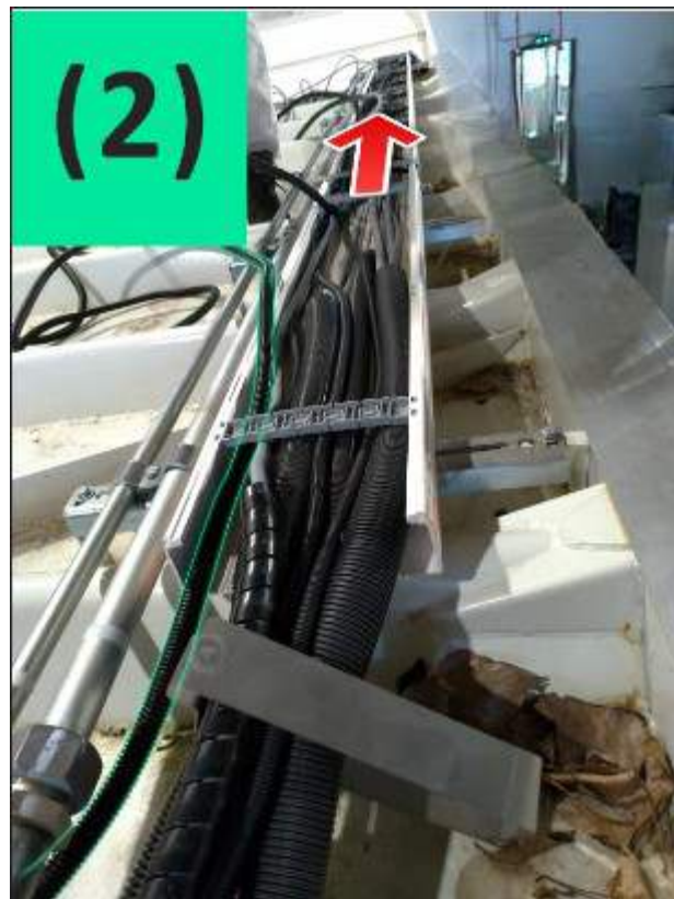
Cable tray on truck roof to cab
