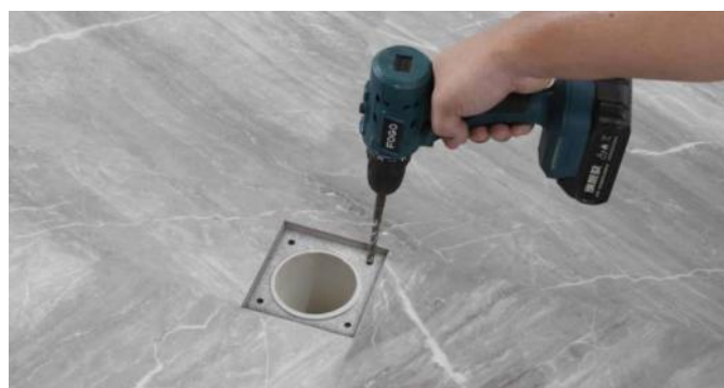
3. Take off the fixed disk and drill four holes for screws.
