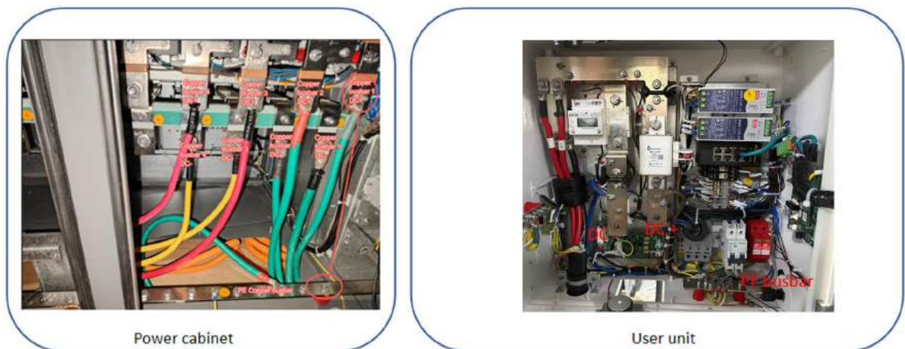
Figure 6-4 Verification of DC Cables
