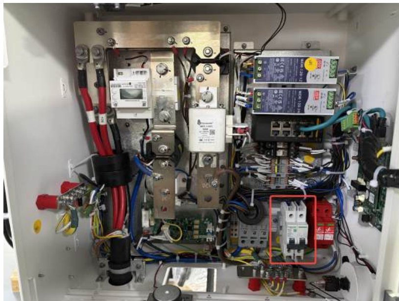
Figure 6-8-1 Turn on the RCCB inside user units
