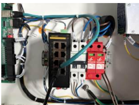
Figure 6-6-2 Switch inside control box
