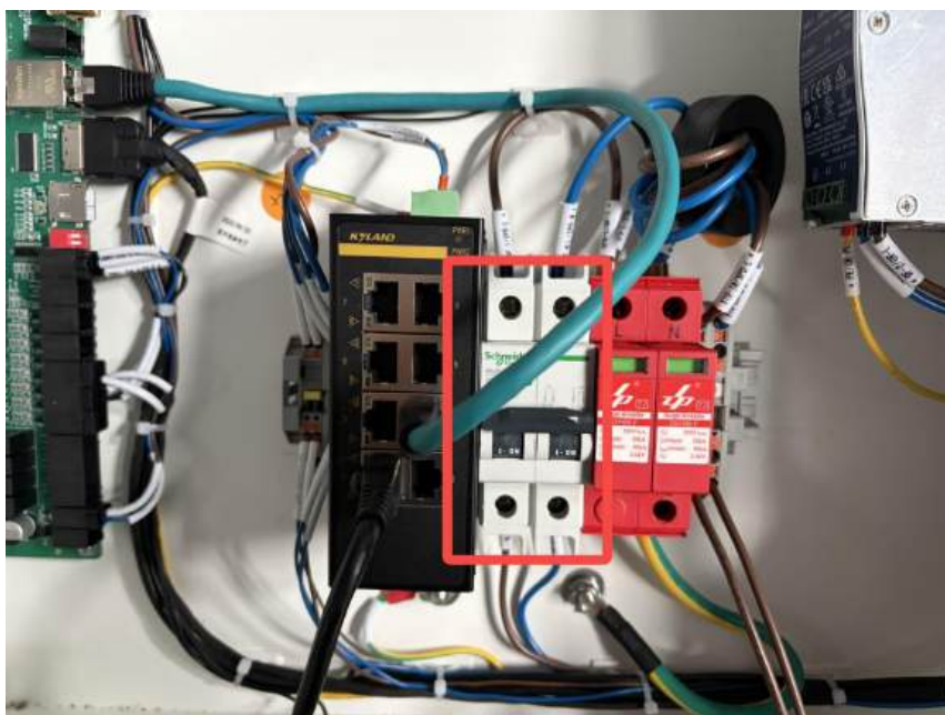
Figure 6-8-2 Turn on the RCCB inside control box
