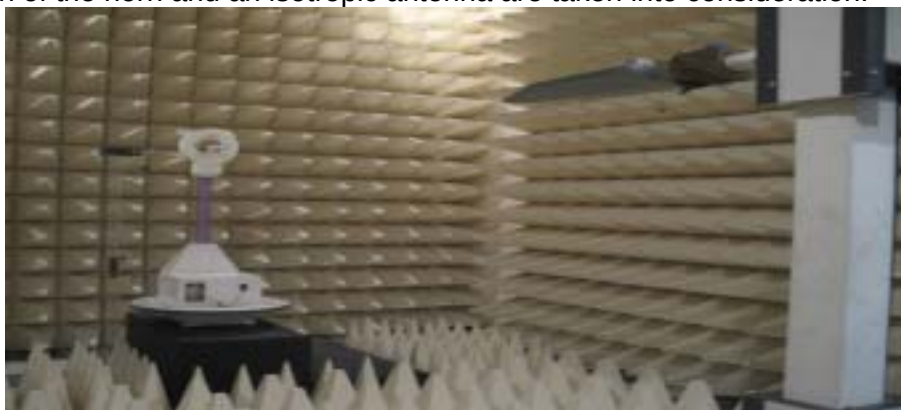
Figure2. Photograph of 3m Fully-Anechoic Chamber
