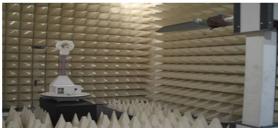
Figure2. Photograph of 3m Fully-Anechoic Chamber
