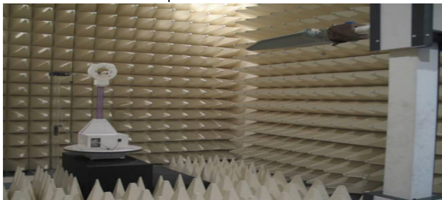
Figure2. Photograph of 3m Fully-Anechoic Chamber
