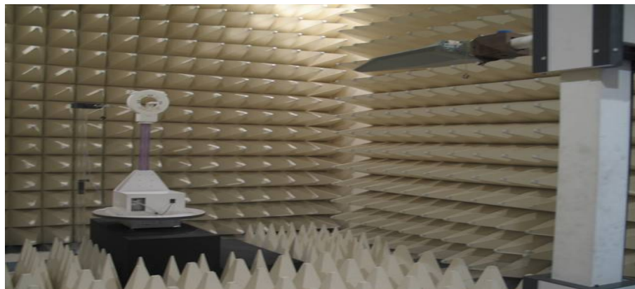
Figure2. Photograph of 3m Fully-Anechoic Chamber
