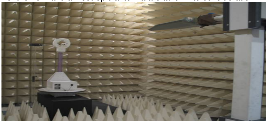
Figure2. Photograph of 3m Fully-Anechoic Chamber
