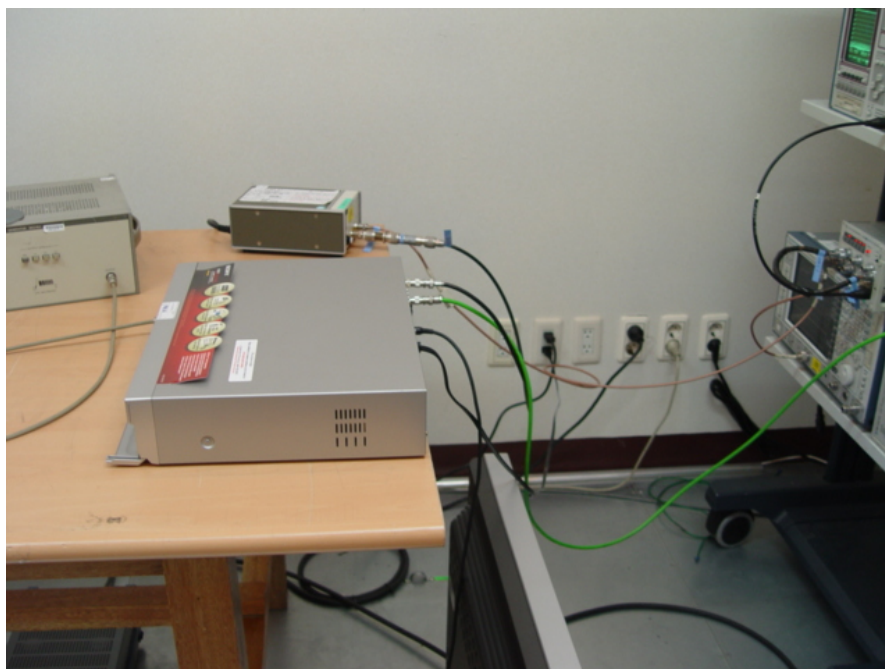
Picture 6. Ant. Transfer Switch
