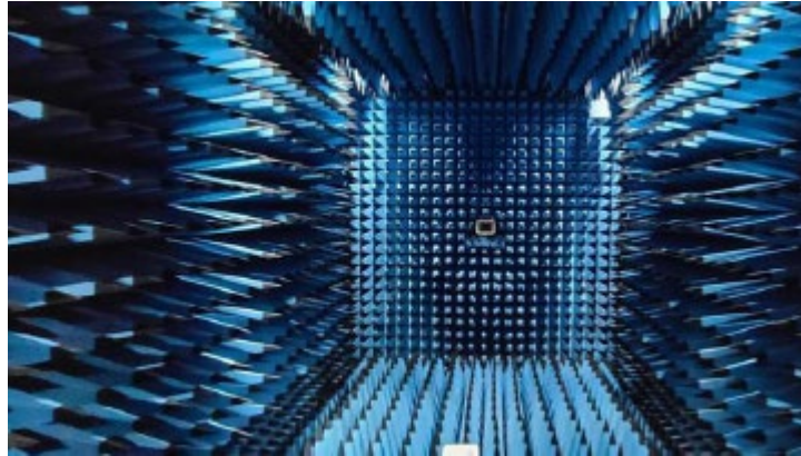
Figure 1: Geometry of Anechoic Chamber for Radiation patterns.
