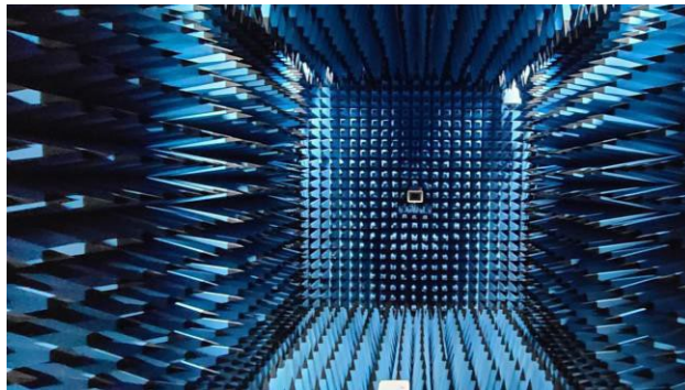
Figure 2: Geometry of Anechoic Chamber for Radiation patterns.
