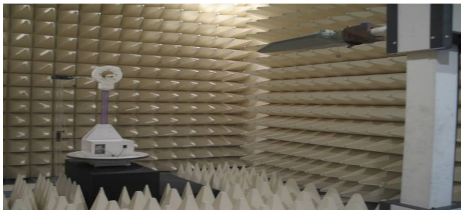
Figure2. Photograph of 3m Fully-Anechoic Chamber
