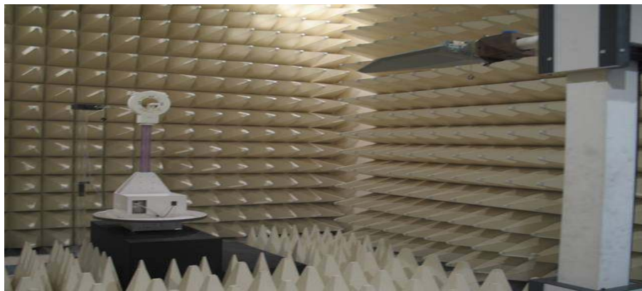
Figure2. Photograph of 3m Fully-Anechoic Chamber
