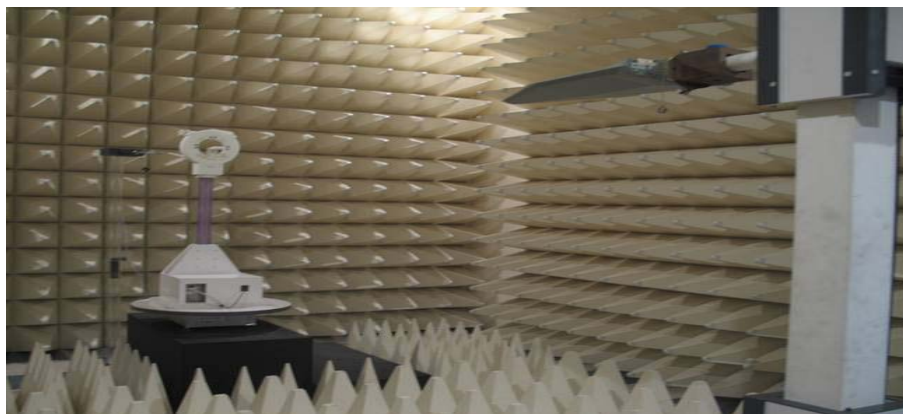
Figure2. Photograph of 3m Fully-Anechoic Chamber
