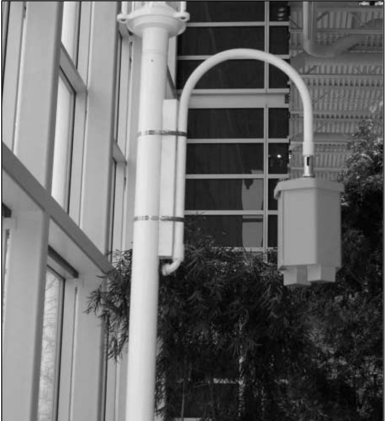
Figure 1-5 AP7220 mounted directly to supporting electrical conduit
