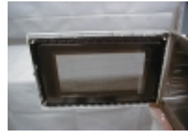
Exhibit 2-H, View of Door Construction Illustrating integral choke
