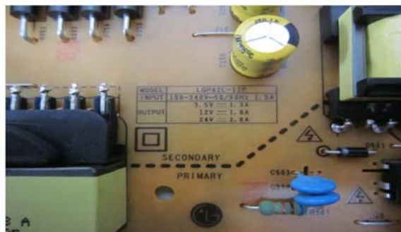
POWER BOARD LABEL(after)
